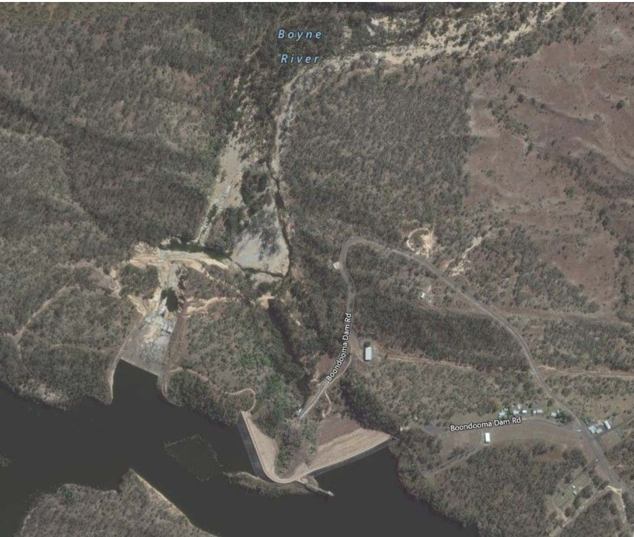
Photo 1: Aerial view of dam and spillway
