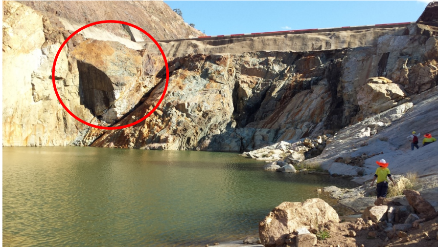
Photo 3: Lower Spillway Chute, wedge highlighted
