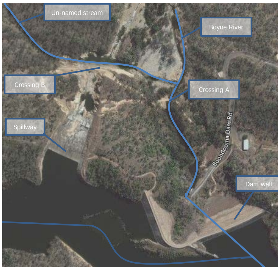
Photo 2: Construction site overview
