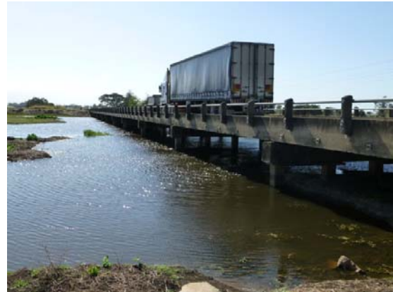
Figure 3 - Existing Cattle Creek Bridge (eastern side elevation)
