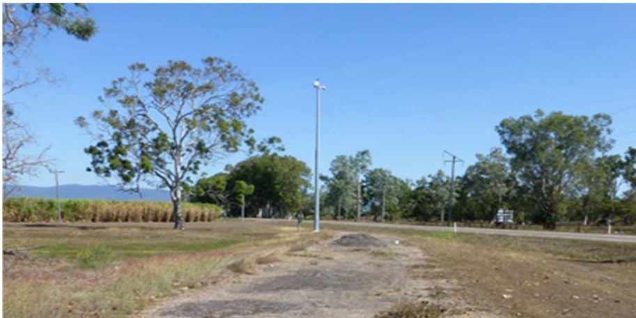
Figure 10 - TMR Camera Pole (at Chainage 111,090m)
