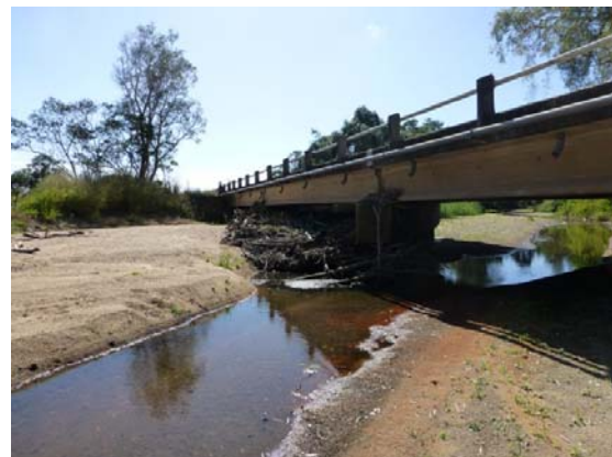
Figure 5 - Existing France Creek Bridge (western side elevation)
