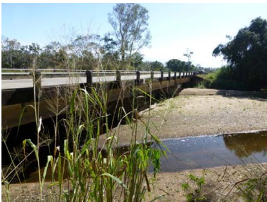
Figure 4 - Existing Frances Creek Bridge (eastern side elevation)
