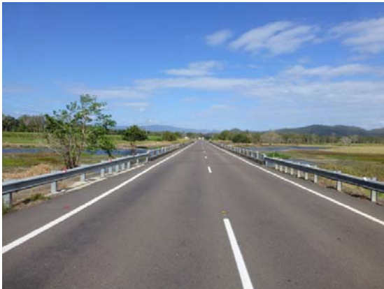
Figure 2 - Existing Cattle Creek Bridge (view looking south)
