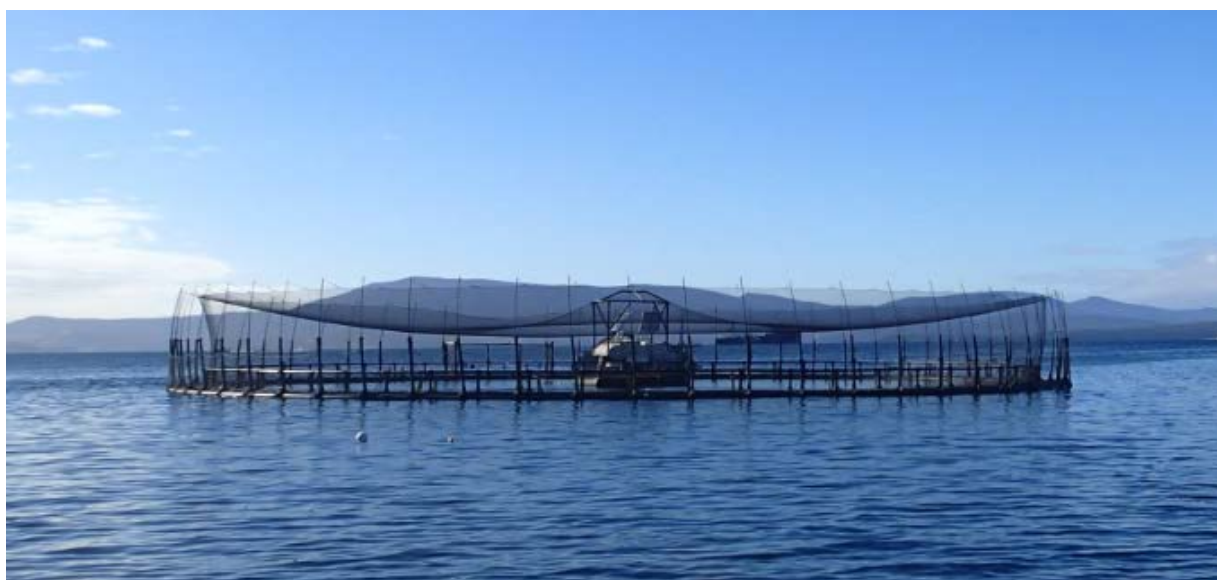
Figure 3: 168m Fortress pen with centrally mounted feed hopper (Source: Huon, 2015).
