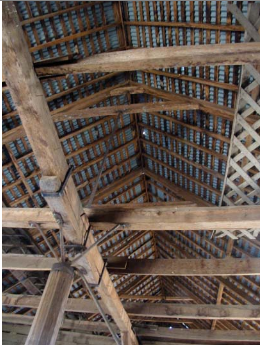
Exposed roof truss framing and shingle battens (Space G01)
