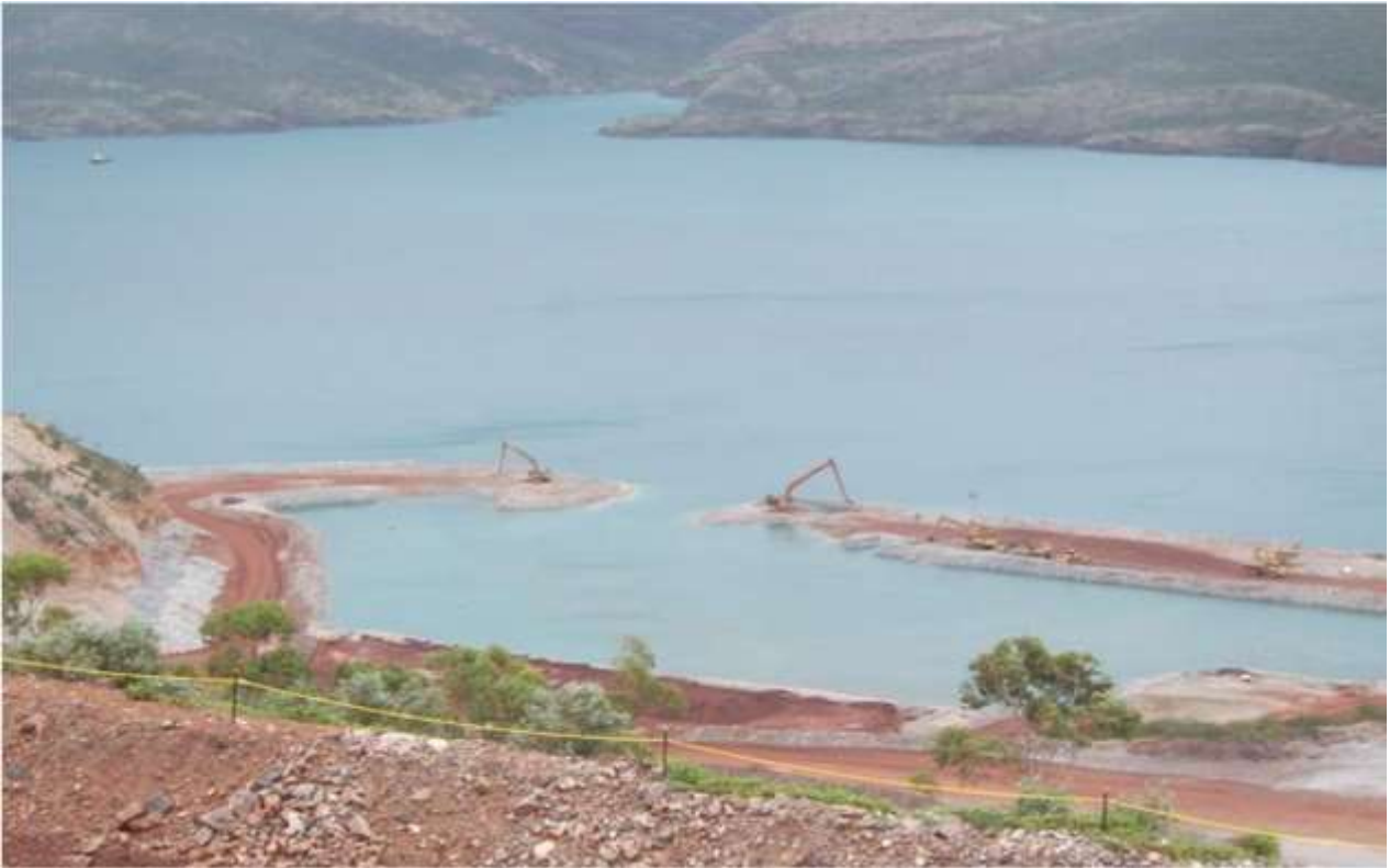
Plate 1: Arbitration Cove Seawall Starter Embankment construction using longreach excavators (looking from Koolan Island across The Canal to the mainland, circa 2008) Source: GHD, 2014
