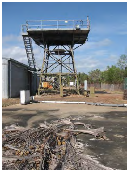
One of the two towers and concrete slab floor foundation
