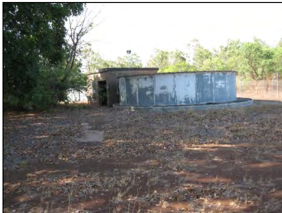
Water tanks and pump house
