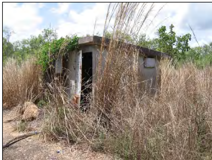
Concrete hut facing southeast
