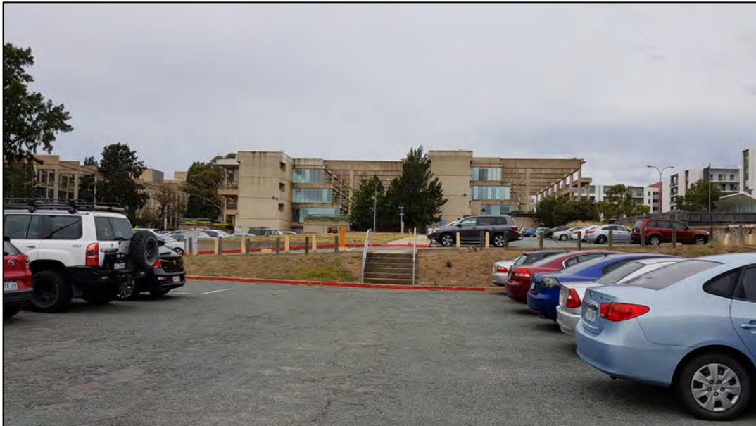
Photograph Three. Western end of Wings 4 and 5 viewed from Block 11 Section 44. The galley beams and columns over the former Courtyard Four.
