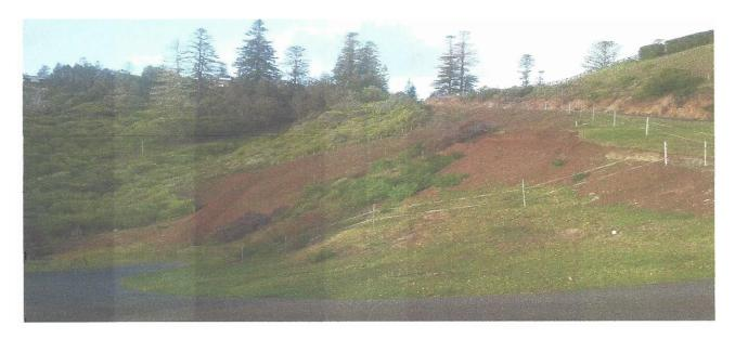
Earthworks include extension of the existing access onto the land constructed along the contour to the proposed dwelling, and excavation for siting of two water tanks, septic tank and an absorption trench. Retaining walls, fill and excavations are to engineer assessment and specification.
