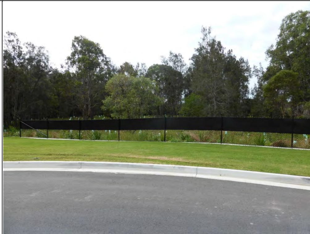
Figure 8: one-way koala fencing at the interface between Gainsborough Greens Development and the koala conservation area (Location 1)
