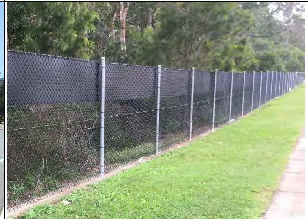
Figure 11: One-way exclusion fencing along northern side of Yawalpah Road (Location 3)
