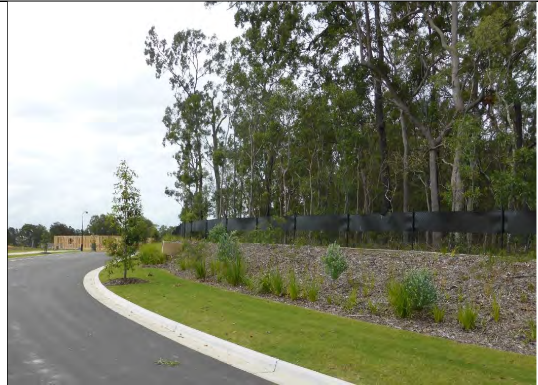
Figure 9: one-way koala fencing at the interface between Gainsborough Greens Development and the koala conservation area (Location 1)
