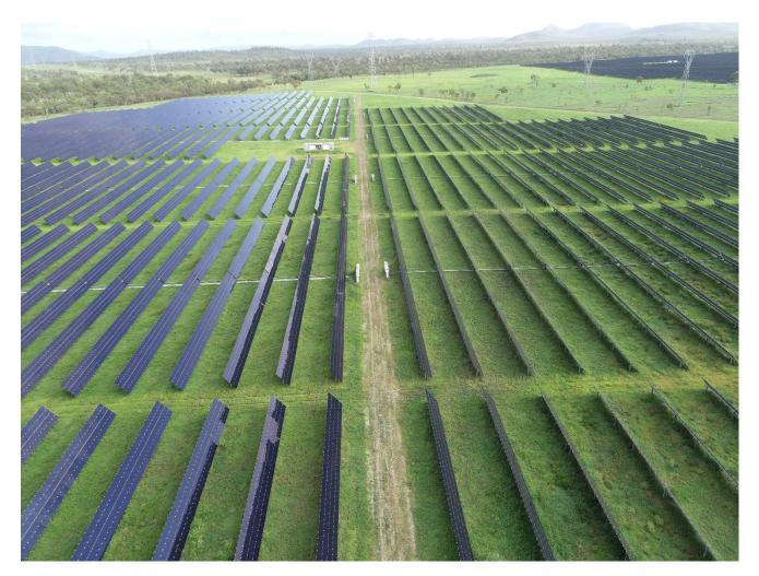
The solar module frames and inverter stations will be installed on piles and sit above ground level. This ensures retention of existing grassland vegetation and habitats in situ with a minimal level of ground disturbance. Regrowth of vegetation will be enabled following temporary disturbance during installation.
