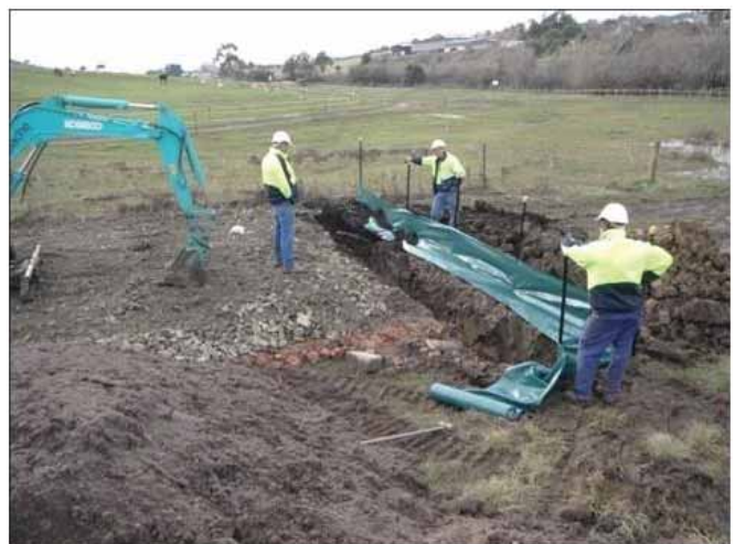
Sump to drain cleandown effluent
