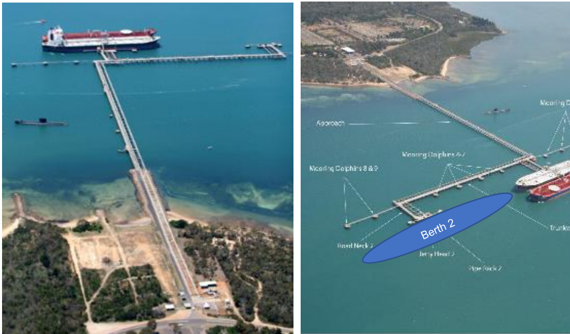
Photo 1: View of Crib Point Jetty from the west Photo 2: View of Crib Point Jetty from the south-east
