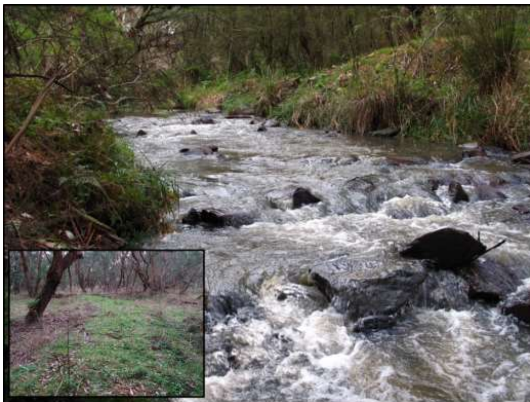
Figure 6. Rockworks placed into Cockatoo Creek in Yellingbo Nature Conservation Reserve ~2000 to prevent upstream progression of head cuts resulting from stream deepening and channelisation. The inset shows the levee constructed along the right-hand bank of Cockatoo Creek in the 1950s. Photographs taken May 2016 by Paul Boon
