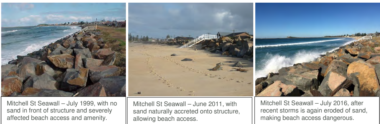
Figure 2-3 Stockton Beach Mitchell St Seawall and Recession over time
