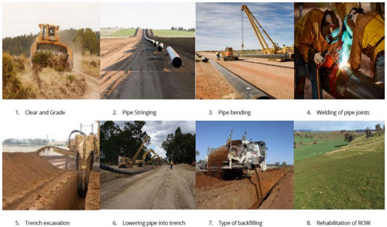
Figure 1. Typical construction sequence
