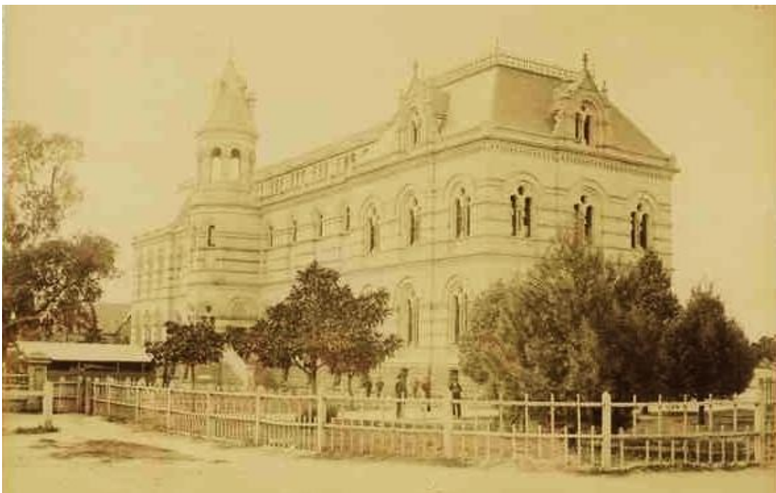
Figure 111 Public Library, west wing, North Terrace, c.1884 Source: State Library of South Australia
