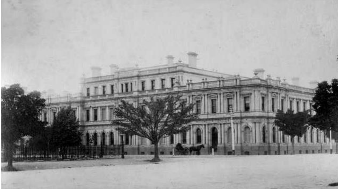
Figure 110 Government Offices, Victoria Square, Michael Egan, 1879-81 Source: State Library of South Australia
