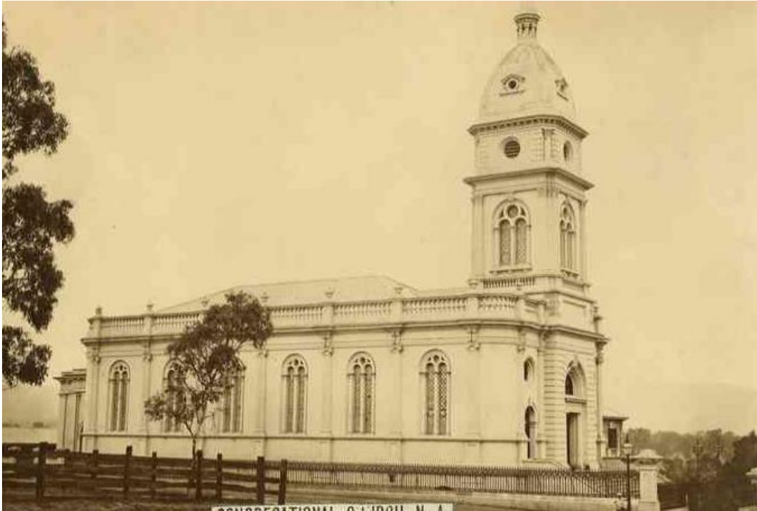
Figure 103 Congregational Church, Brougham Place North Adelaide, after tower added in 1871 Source: State Library of South Australia
