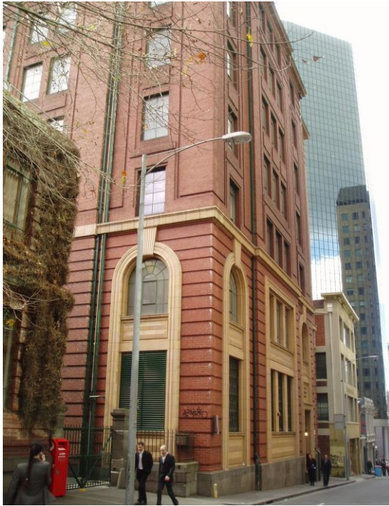
Figure 115 City West Telephone Exchange, Melbourne
