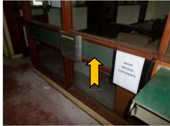
Photo 2. Section 34 – Administration Building, ground floor, room 3 (corridor), infill panels – asbestos fibre cement sheet. Sample: 17069-001-010.
