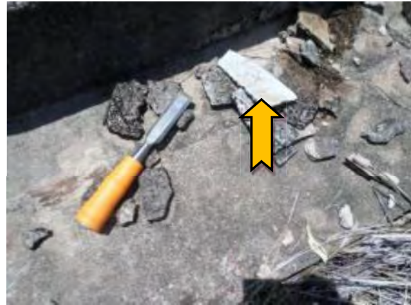
Photo 14. Section 32 – Area E1, external, inside 32 compound, debris – asbestos fibre cement sheet. Reference: 17069-001-029.
