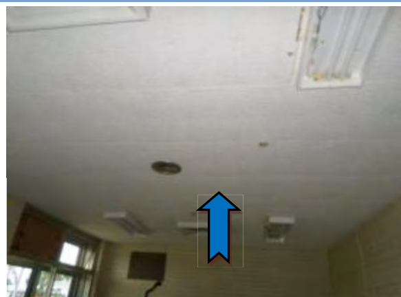
Photo 6. Section 34 – Administration Building, ground floor, room 19 (residents hall, kitchen), ceiling – suspected SMF ceiling tiles.
