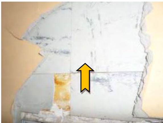
Photo 3. Section 34 – Administration Building, ground floor, room 7 (female toilet), wall lining – grey asbestos vinyl wall tiles. Sample: 17069-001-008.
