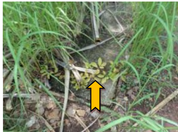
Photo 12. Section 32 – Area E1, external, various locations, service pits – asbestos moulded fibre cement.
