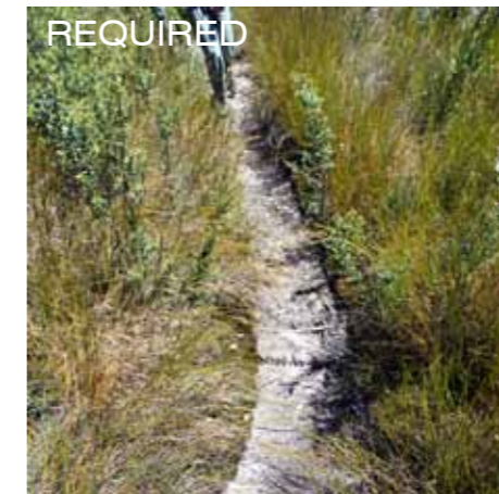
IMG 1829 - Required due to trenching
