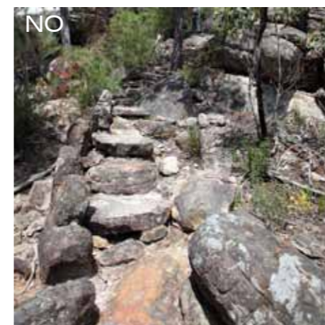
IMG 1622 - Avoid stone edging to main steps
