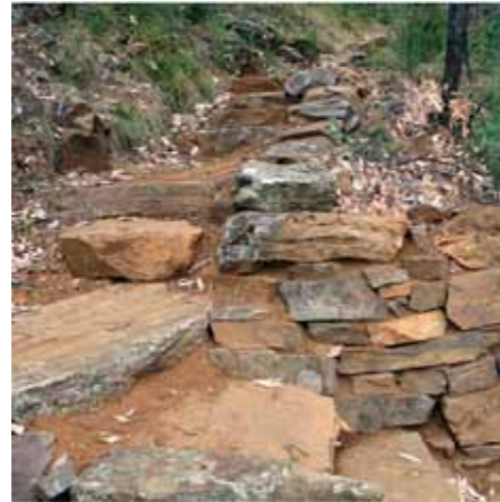
Rock armouring on switchback (Courtesy TTMS)
