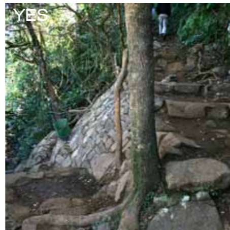
Rock armouring on switchback (Courtesy TTMS)
