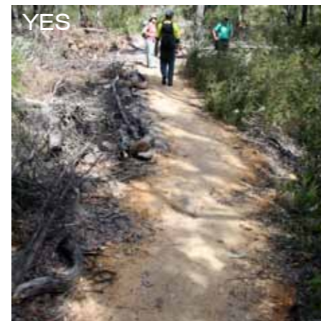
IMG 6669 - Compacted earth water bar
