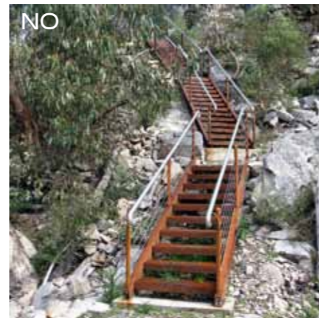
IMG 3671 - Too constructed, dissimilar materials
