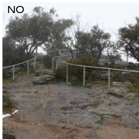
IMG 5830 - Excessive use of oversized railing
