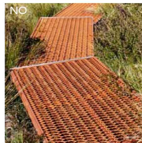
Expanded mesh too harsh / industrial
