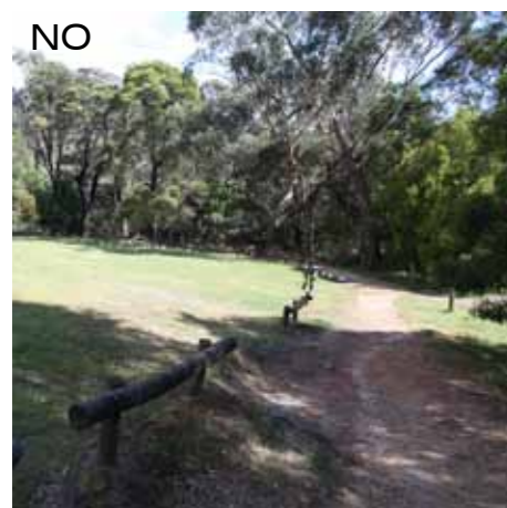
IMG 1518 Poor Access to main Trail from town
