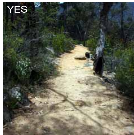
IMG 6623 - Compacted earth water bar
