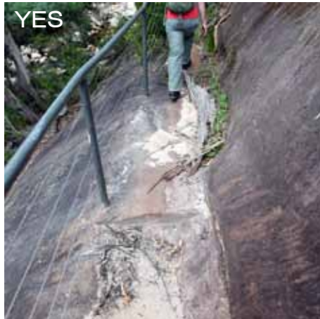
IMG 1552 - Steps cut into existing rock shelf
