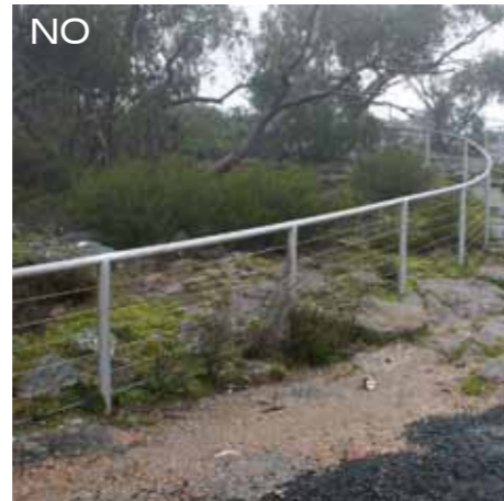
IMG 5831 - Excessive use of handrail
