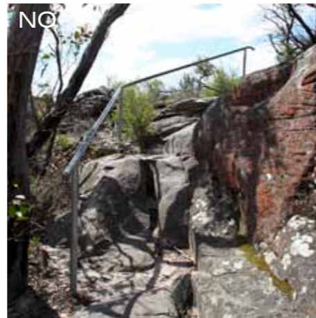
IMG 1737 - Unnecessary handrail
