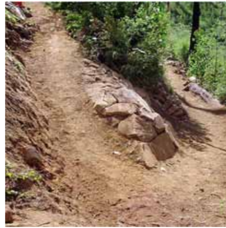
Rock armouring on switchback (Courtesy TTMS)
