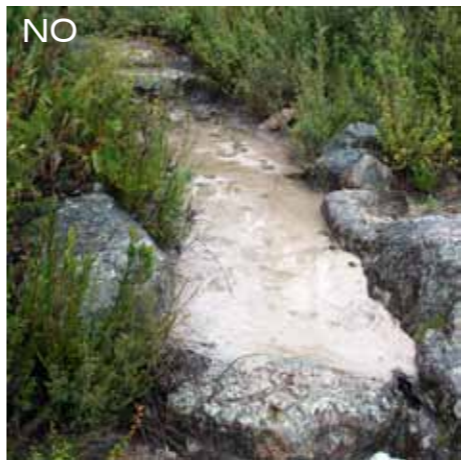
NO IMG 5826 - Poor drainage during rain storm
