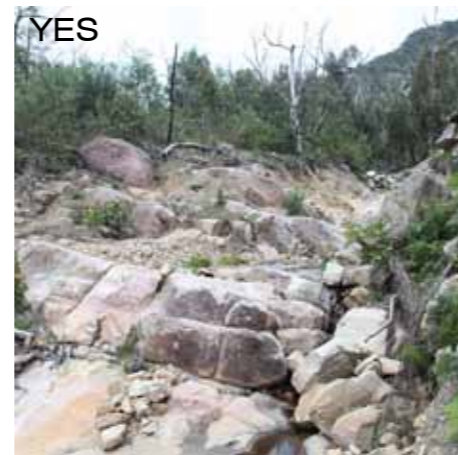
IMG 1570 - Landslip with exposed rock shelf
