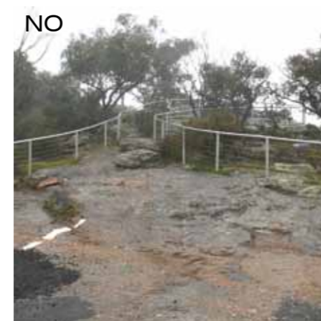
IMG 5830 - Poor interface with carpark (Reeds)
