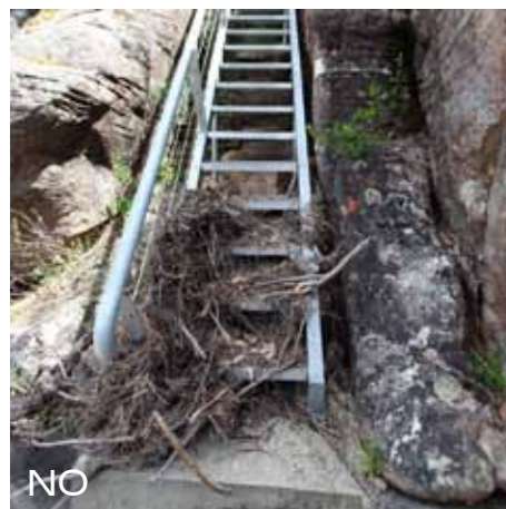
IMG 1611 - Large concrete plinth required
