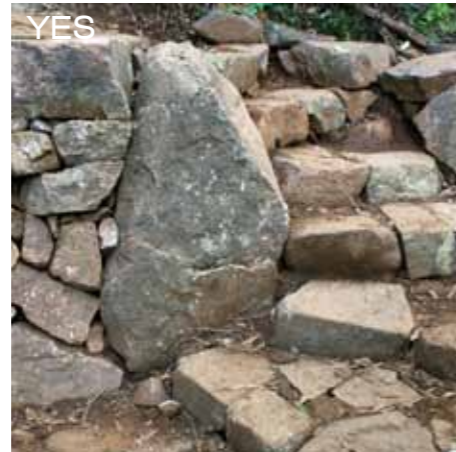
Rock armouring on switchback (Courtesy TTMS)
