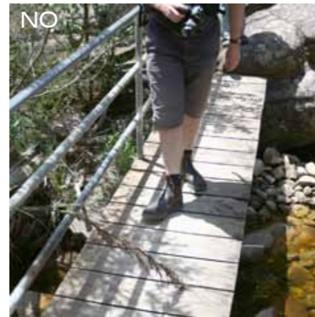
IMG 6595 - Do not use solid steel mid rails
