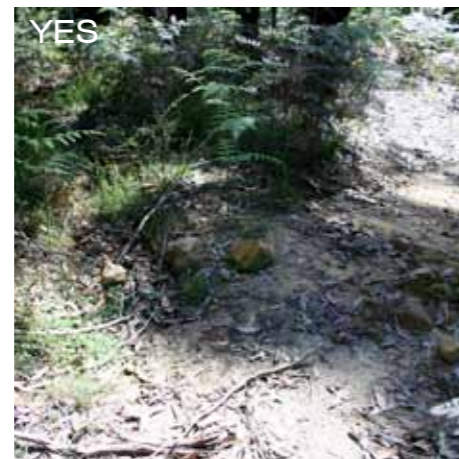
IMG 6686 - Compacted earth water bar
