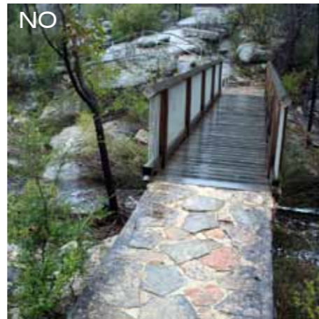
IMG 5805 - Handrail too heavy
