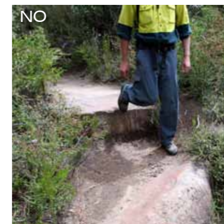
IMG 1569 - Erosion at foot of step
