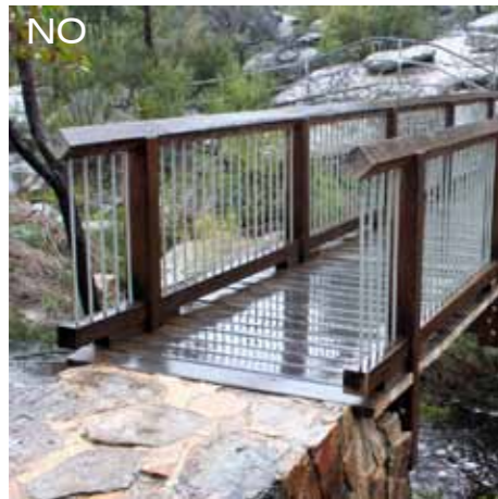
IMG 5808 - Too much steel work,
