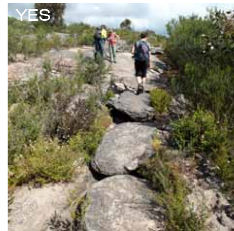
IMG 1747 - Use of large stones to bridge height
