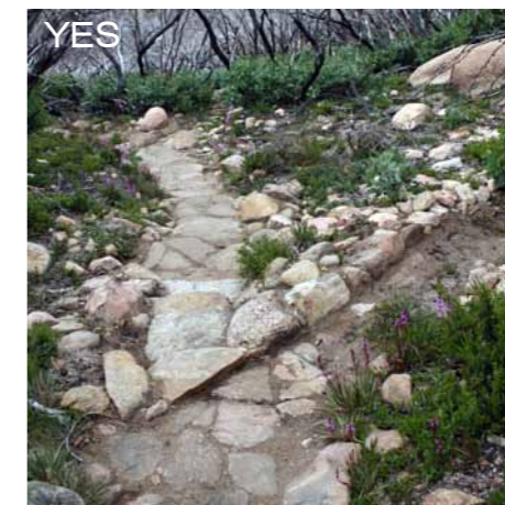
Stone water bar, Mount Buffalo (Courtesy TTMS)
