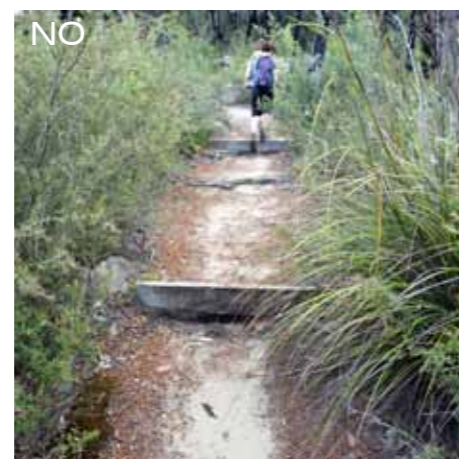
IMG 1765 - Timber steps with erosion
