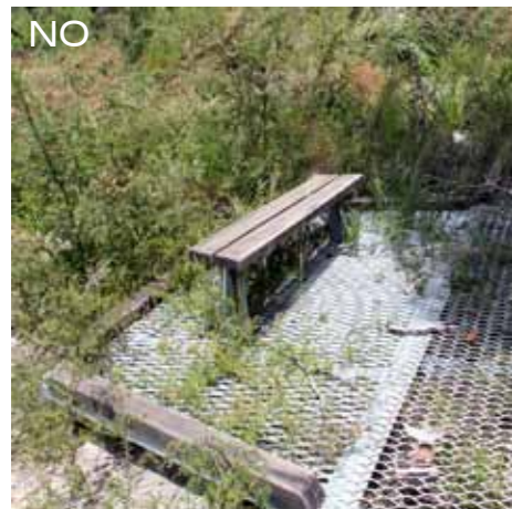
IMG 1667 - Seat too constructed / out of place
