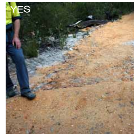
IMG 6676 - Compacted earth water bar
