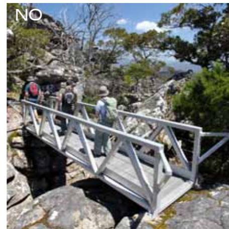
IMG 1876 - Too bulky (fully prefabricated)
