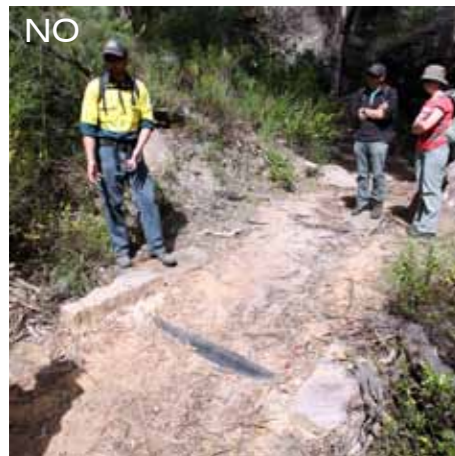
IMG 1524 - Do not use pipe or culvert
