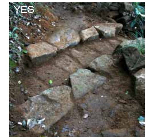
Stone water bar, Mt Warning (Courtesy TTMS)
