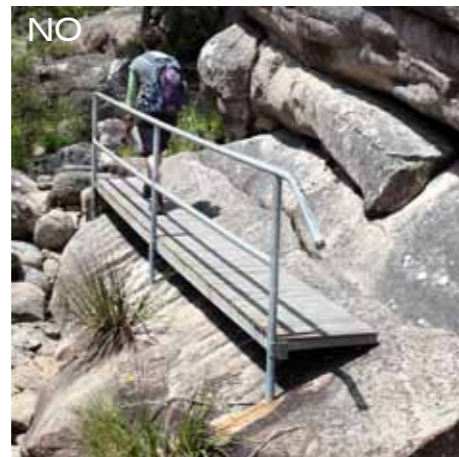
IMG 1633 Awkward trip hazard
