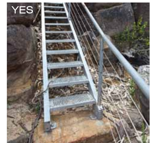
IMG 1606 - Stone plinth at base is good
