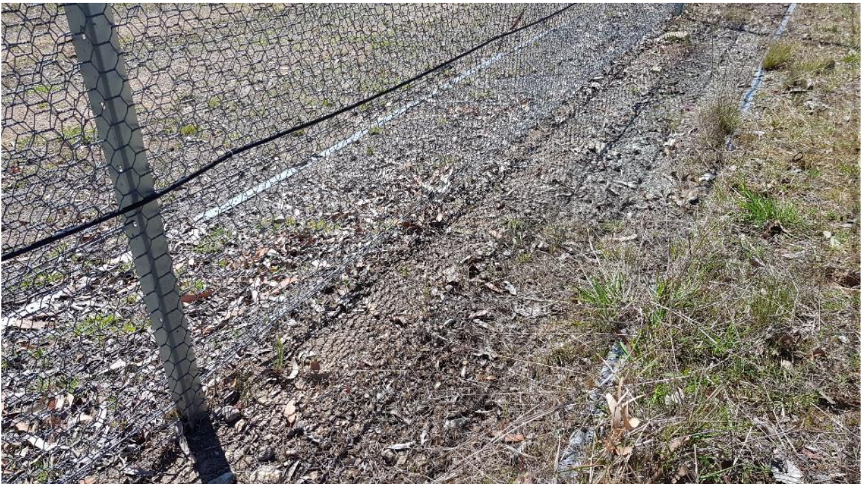
Plate 2. Existing Mulligans Flat Woodland Sanctuary fence – illustration of mesh extending out each side of the fence base.
