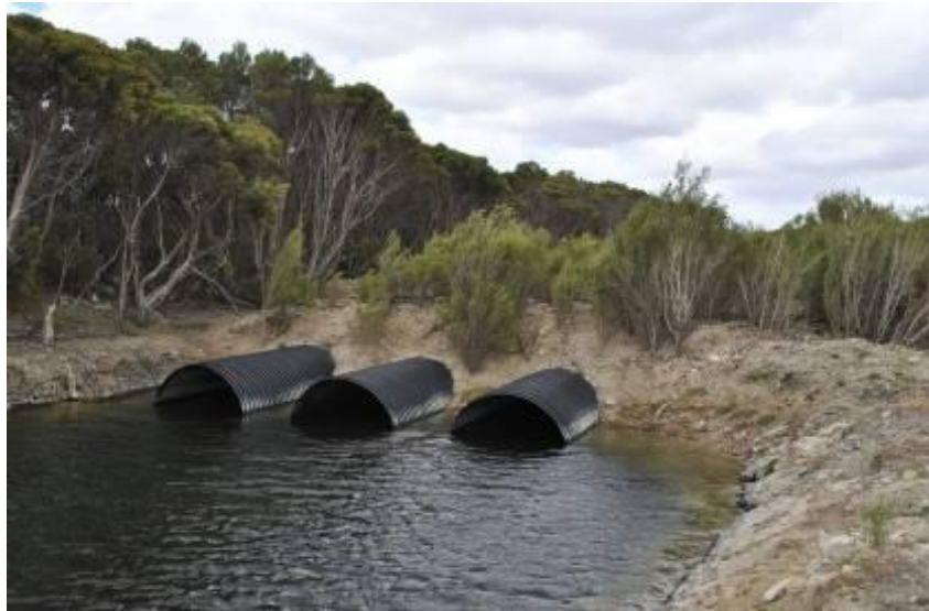
Figure 14: Tilley Swamp drain fauna crossing (R. Seaman)
