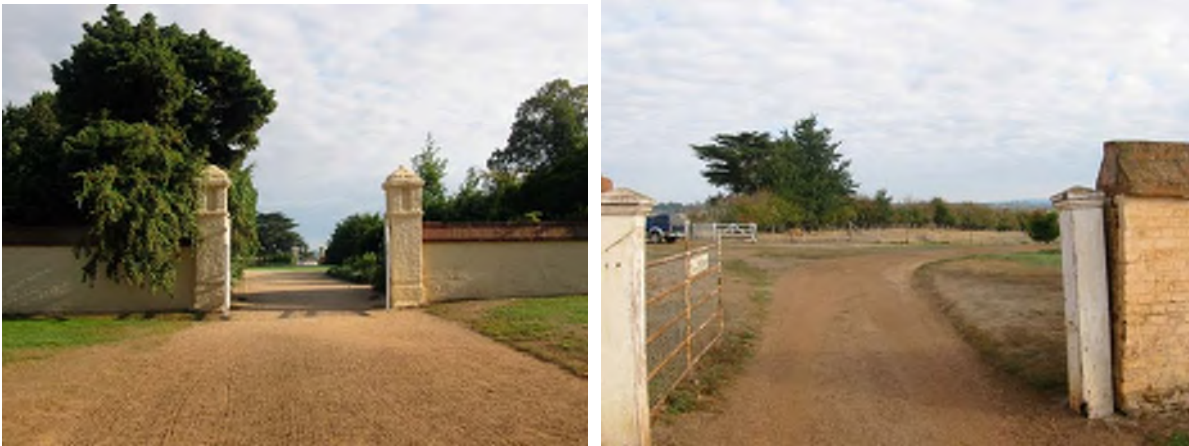
Figure 3. 2: (Left) Roughcast brick gate posts in the garden wall. (Right) Timber capped gate posts in the coach house precinct.
